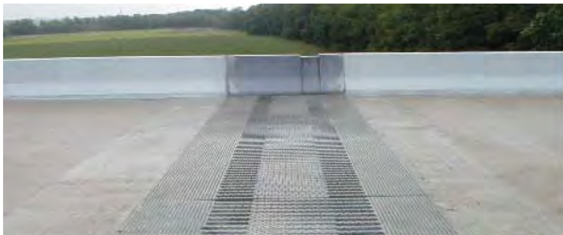
Expansion joints allow bridge sections to expand without breaking.
