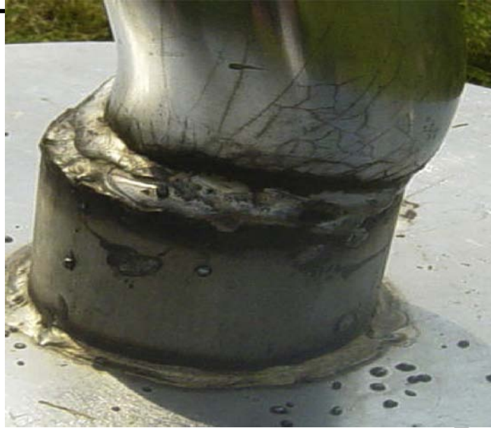
Stress corrosion cracking of austenitic stainless steel
