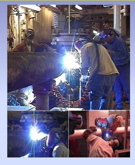
The various pipe sections are then welded together into one continuous length, using manual, semiautomatic or automatic welding procedures.
