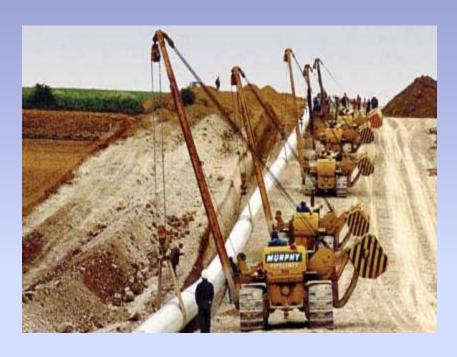
Once the pipeline is welded and coated, it is lowered into the trench. Lowering is done with multiple pieces of specialized construction equipment called sidebooms.
